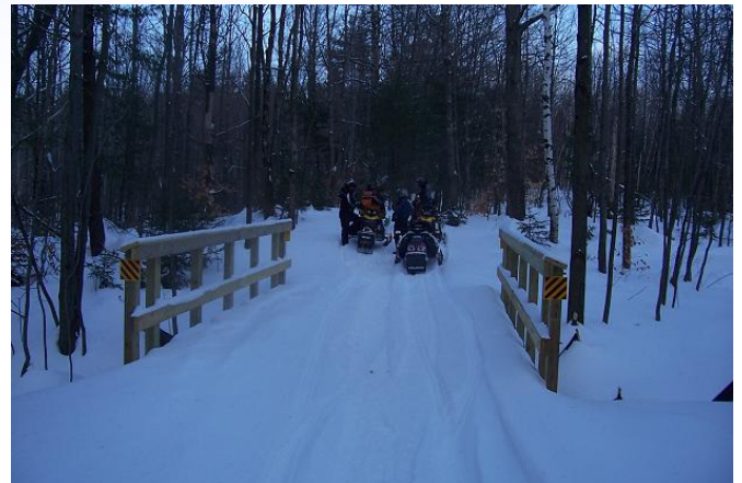
Newly built DEC bridge on Trail C7F in the Charleston State Forest, Burtonsville.
