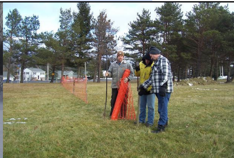
Brian, Matt and Rich install snow fence near Duanesburg Elementary.
